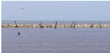
Figure 1.3 Construction of a Sea Wall or Breakwater at Tanjung Senekip Beach
